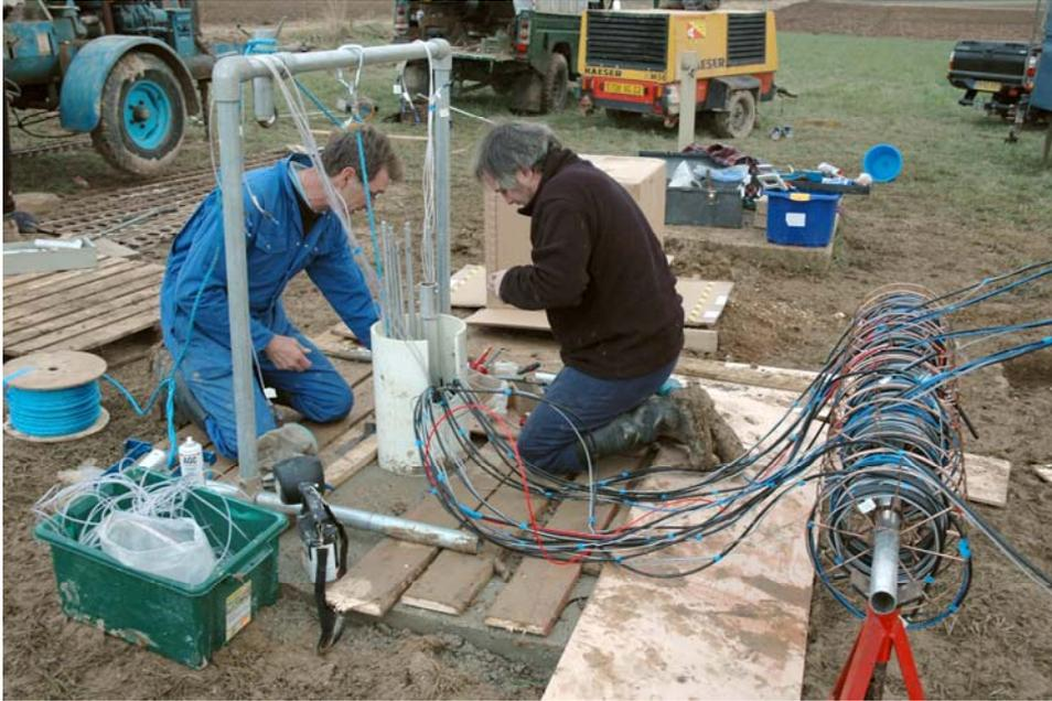
*Figure 1 - Installation of the jacking-tensiometers in P6 borehole at Warloy-Baillon, with assistance of the CEH staff*
